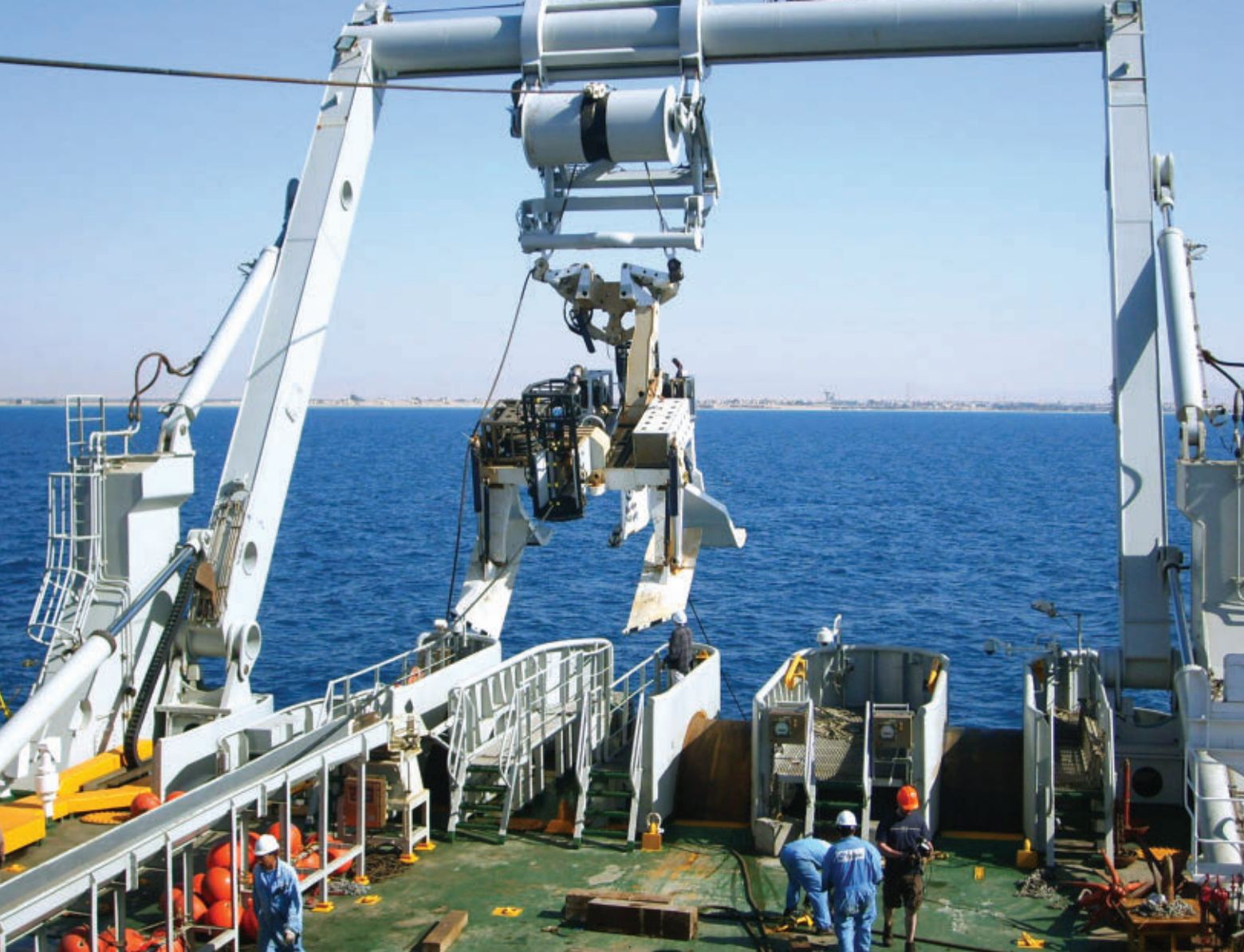
In shallow waters, cable is buried using remotely operated sea plows. Here, a sea plow is loaded into the sea. In the background is Ras Sidr, Egypt. Courtesy of Tyco Telecommunications.
