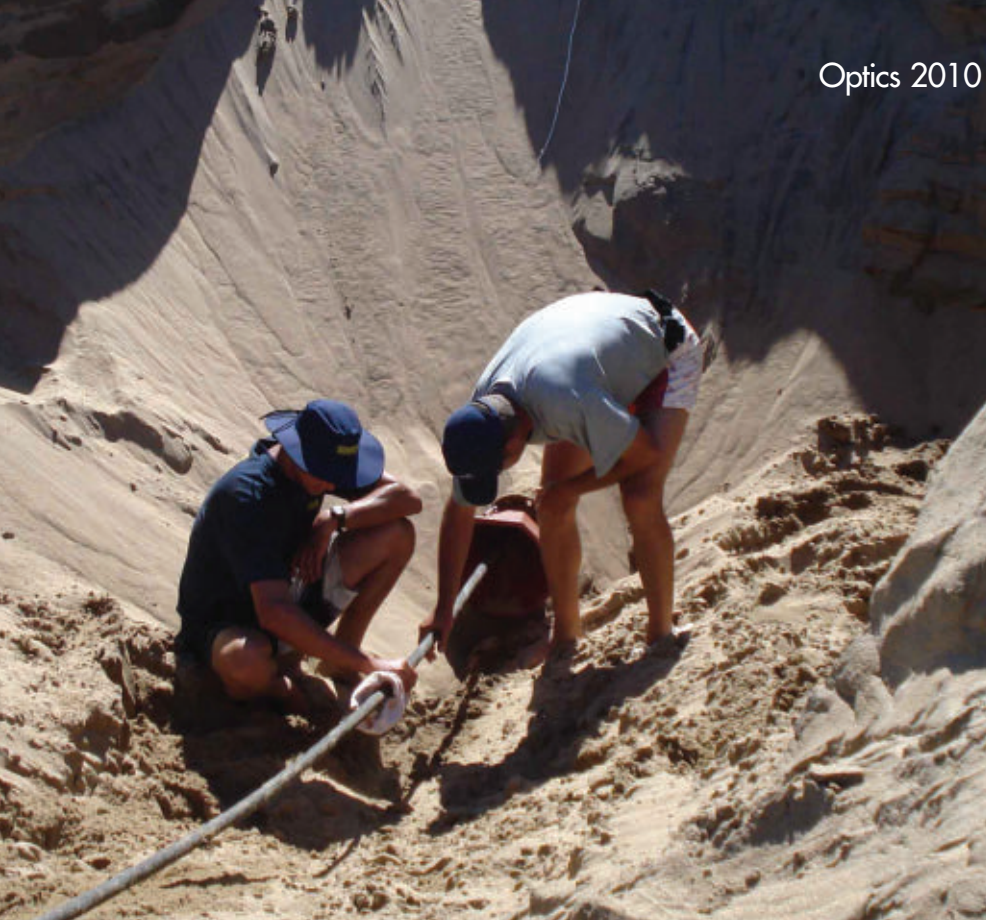
Seacom's pull-through bore pipe helps engineers bury the cable underground. Courtesy of Seacom.
