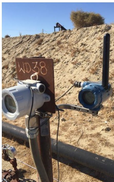
Wireless totalizers were connected to existing turbine flow meters in five minutes, and were communicating with the control system five minutes later.
