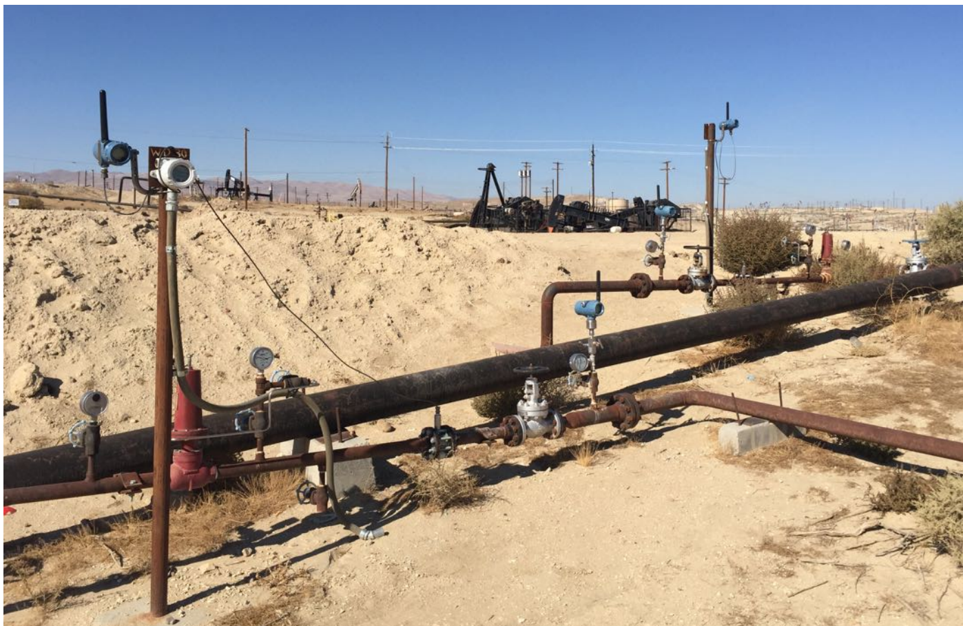
Wireless pressure and totalizing transmitters were installed on 15 water disposal wells.
