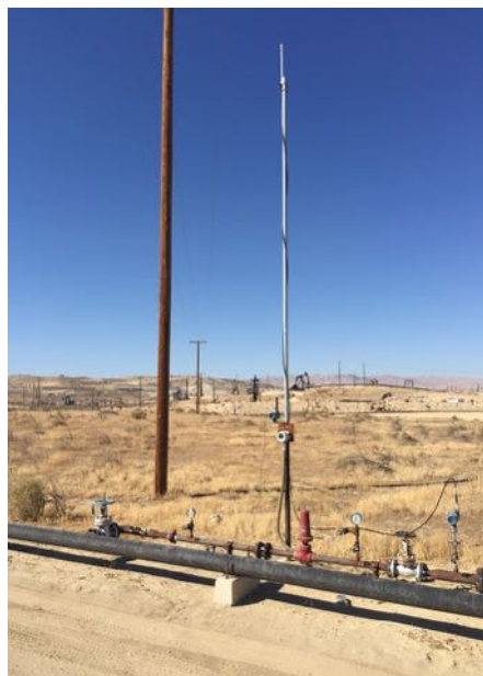
High gain antennas are used when long distances are required for wireless transmissions.
