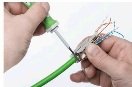
Fastening the casing with a screwdriver
