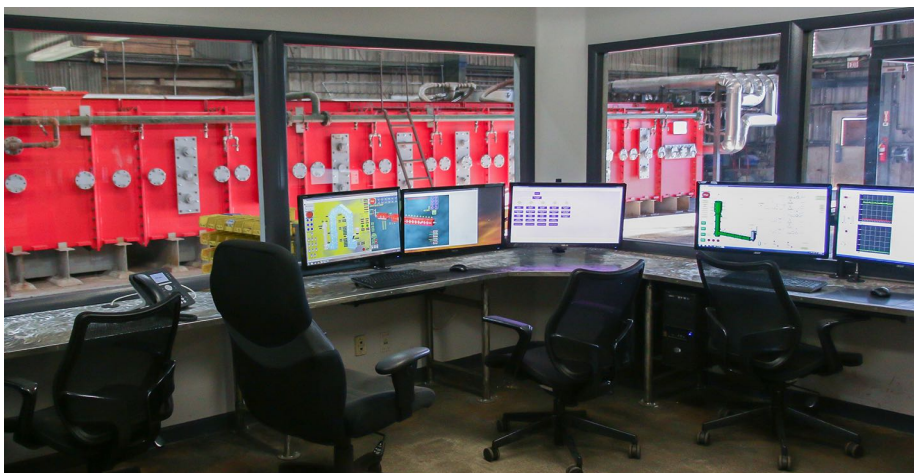
All operations of process equipment at ICGRS can be monitored and controlled from this central control room.
