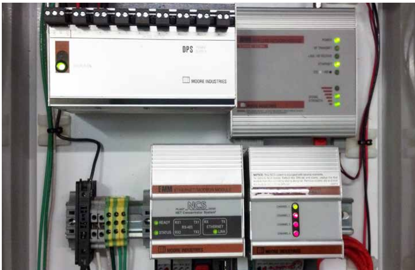
The wireless receiving panel installed at the boiler room of the pulp and paper mill. An EMM Ethernet/MODBUS Interface Module of the NCS NET Concentrator System served as a MODBUS Master to retrieve HART data from the HCS at the pond site.
