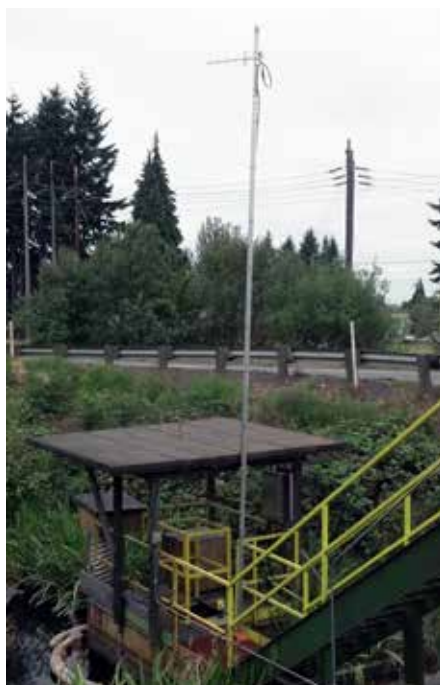
The Yagi-directional antenna was used at the pond site to transmit level signals from the HART level transmitter to the boiler room.
