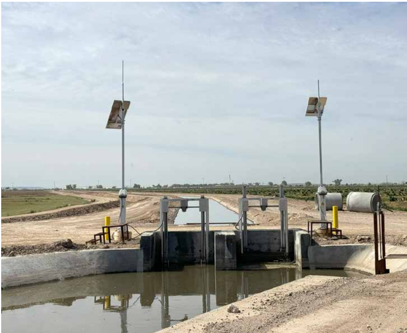
PIDD solar-powered, automated control gates.
