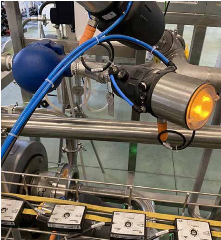
groov EPIC also integrates the Water for Injectables (WFI) plant using ASI bus.
