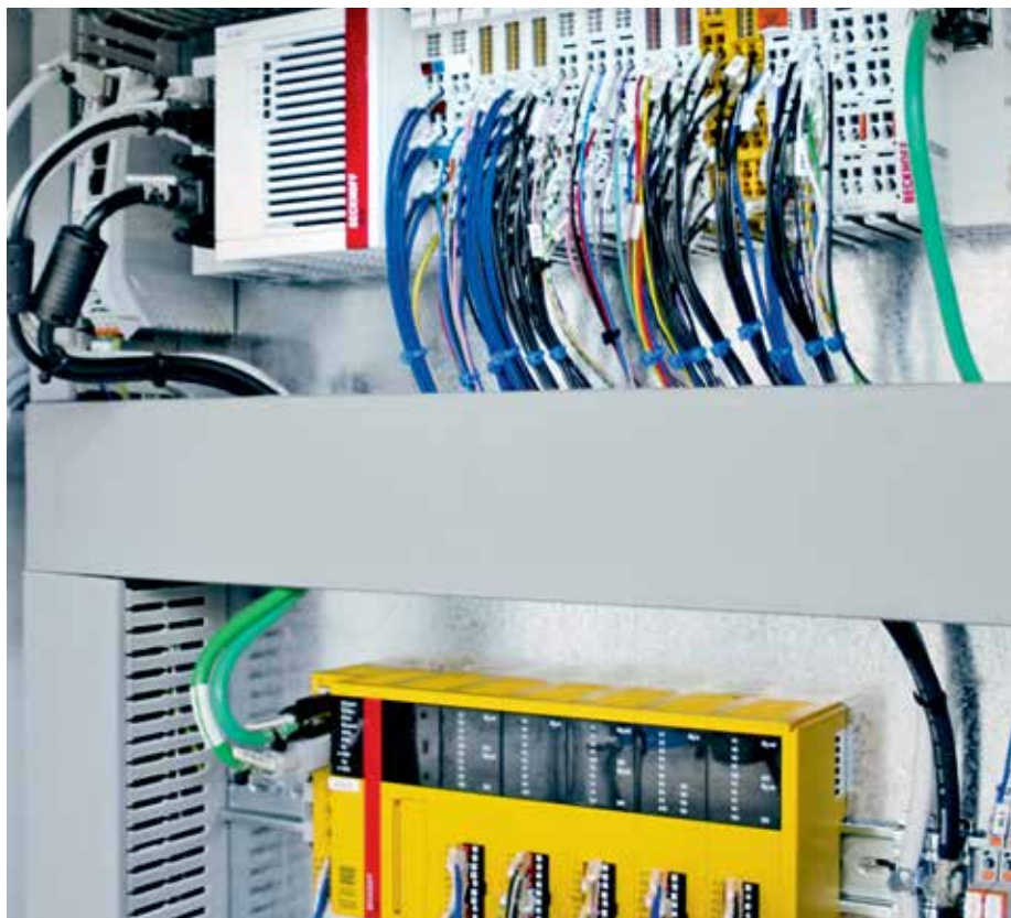
Borgi implements the safety functions with the EK1960 TwinSAFE Compact Controller (below) and additional TwinSAFE terminals, which are integrated into the upper EtherCAT Terminal segment and directly connected to the CX2040 Embedded PC.
