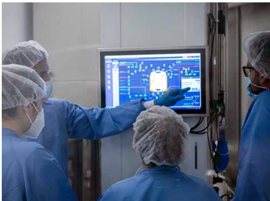
groov EPIC also integrates the Water for Injectables (WFI) plant using ASI bus.
