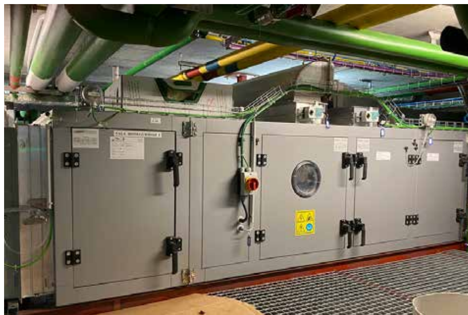
Air Handling Units (AHU) guarantee sterile conditions inside production areas.
