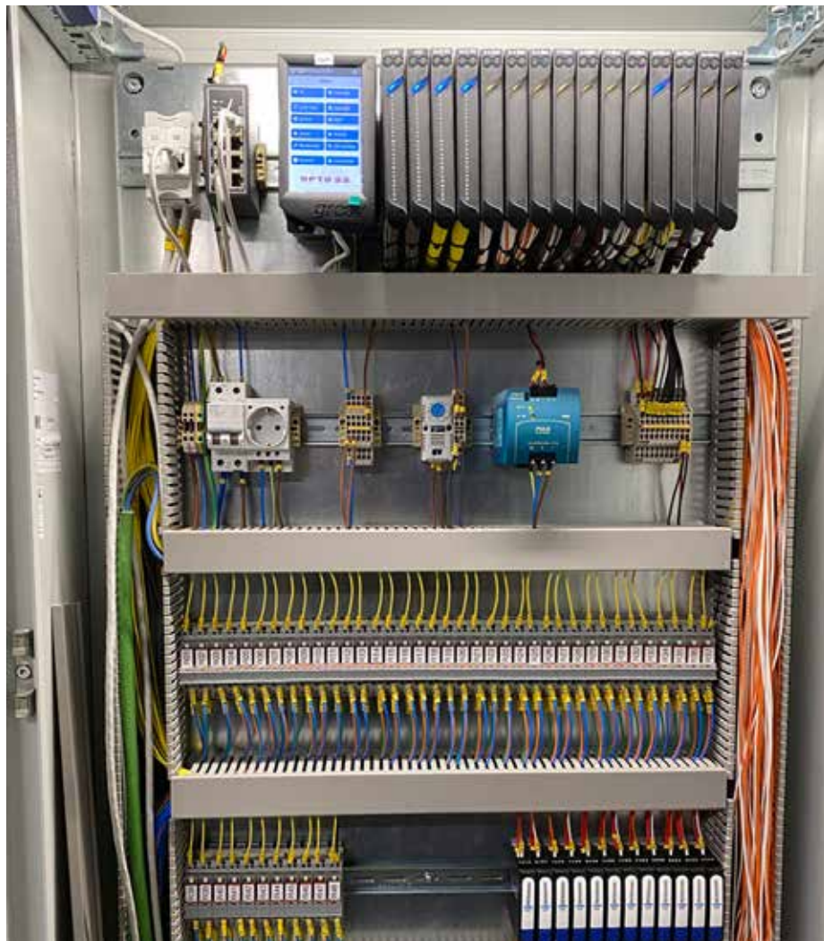
One of the many groov EPIC distributed control system cabinets.
