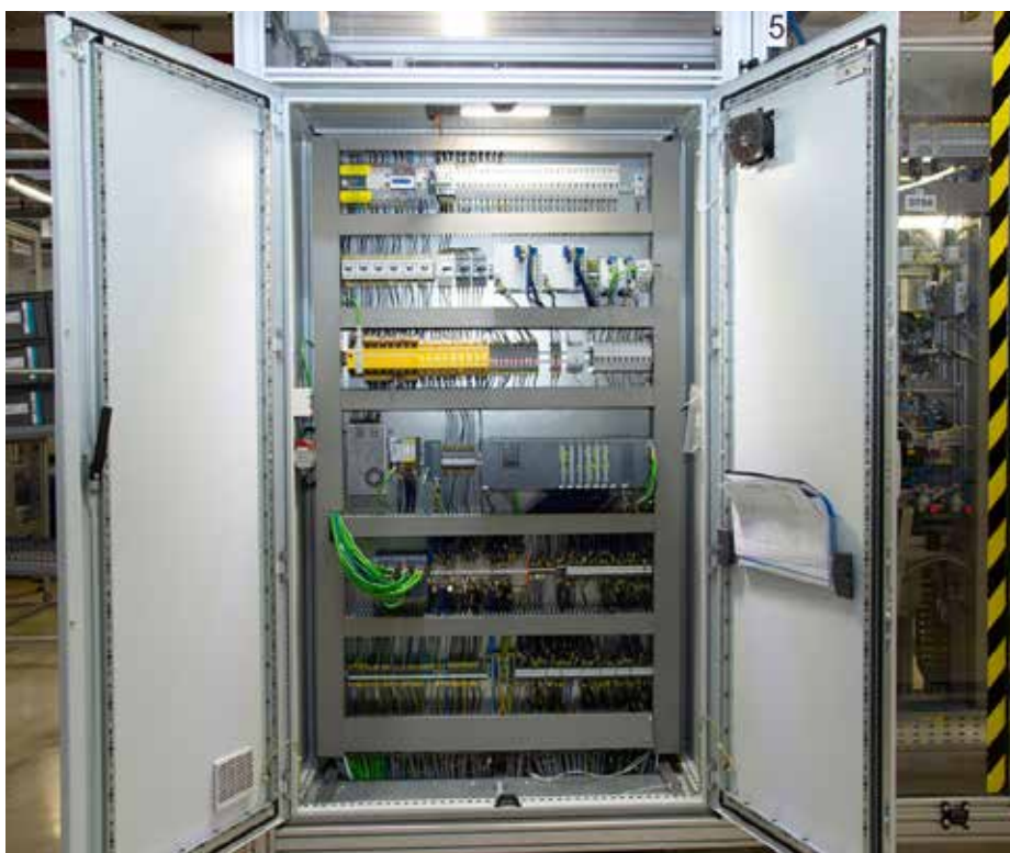
Switchboard with connected Scalance S615 for higher cybersecurity for each production line.
