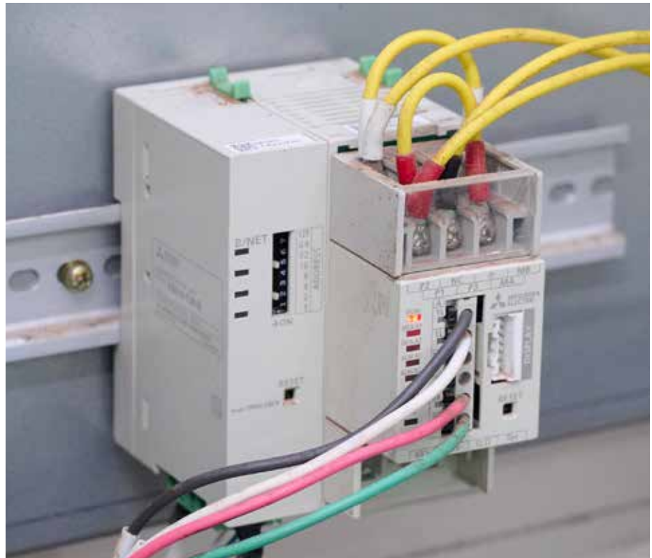
EcoMonitorPlus" installed for demand monitoring.
