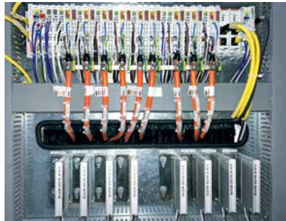
The EL72x1 servomotor terminals (top) and the compact ZB8110 brake resistors (bottom) make for a space-saving control cabinet design.
