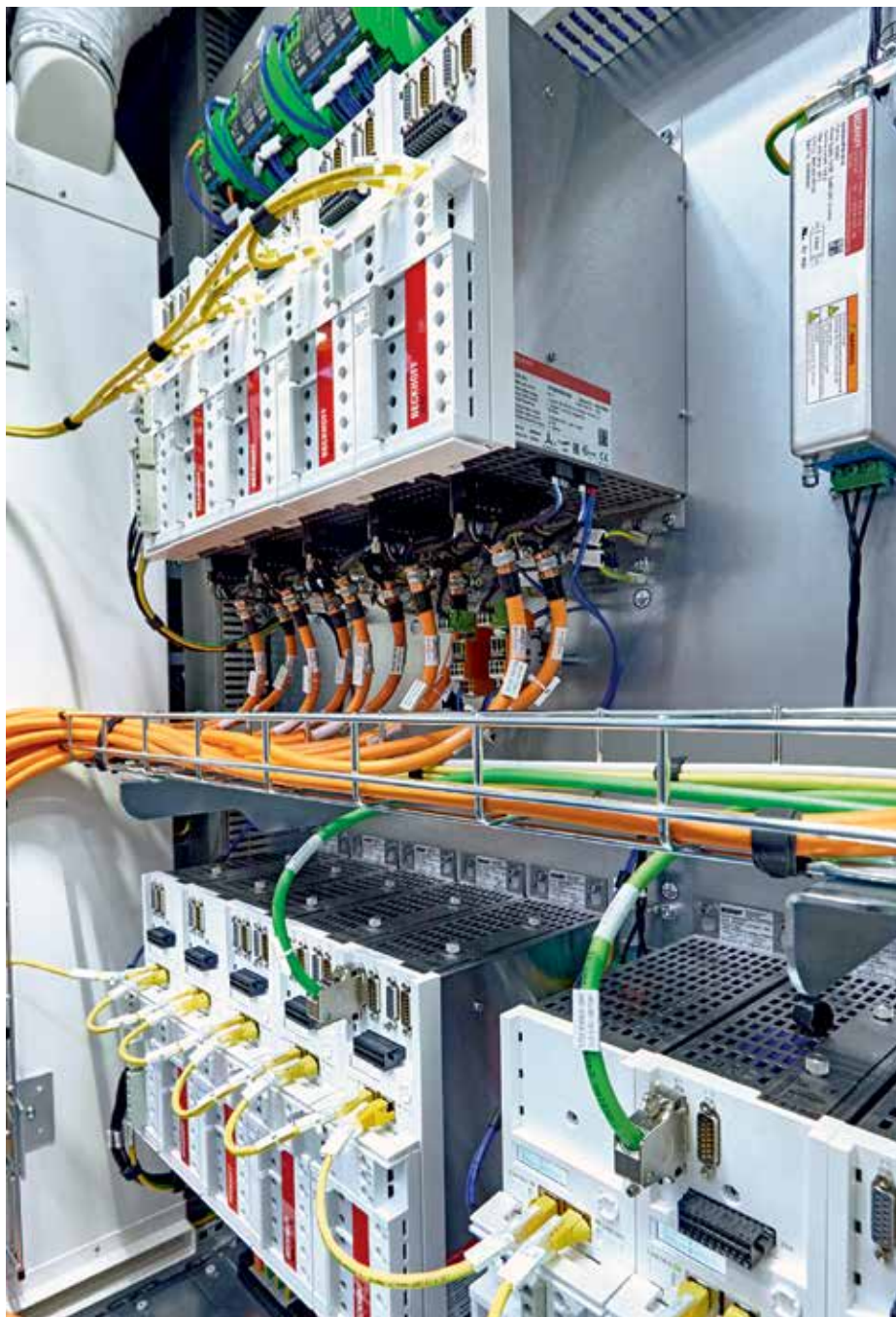
In addition to the compact drive technology, AX5000 Servo Drives are primarily used to control the AM8000 servomotors, with One Cable Technology (OCT) for minimization of installation space and cabling effort.
