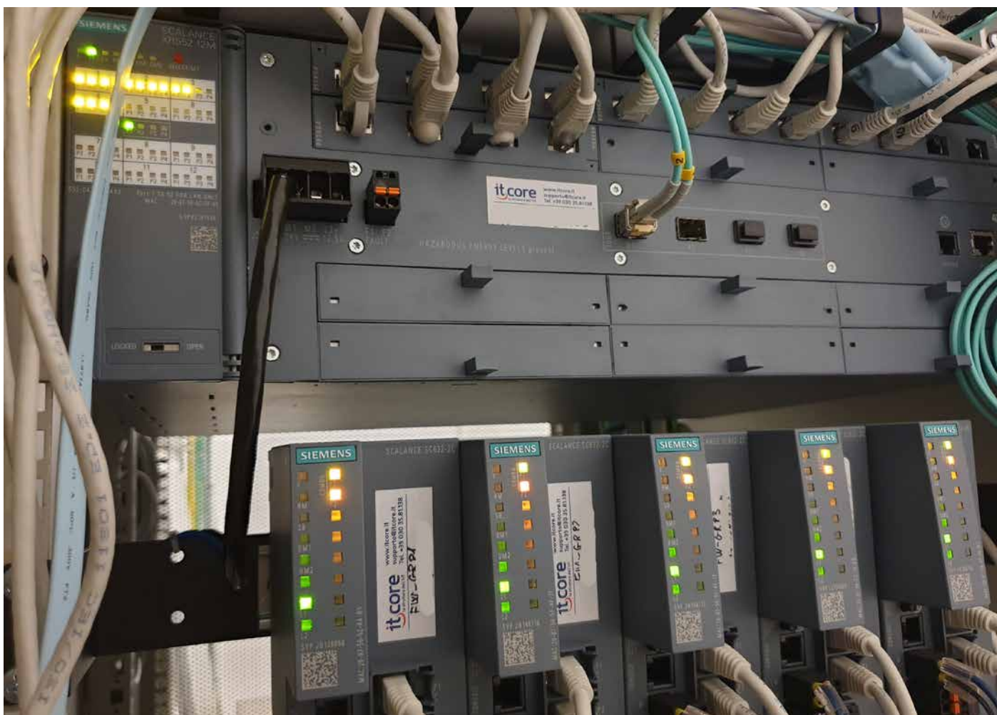
Scalance SC632: the array of industrial firewall enables the right communication path from plant network to IT and vice versa.
