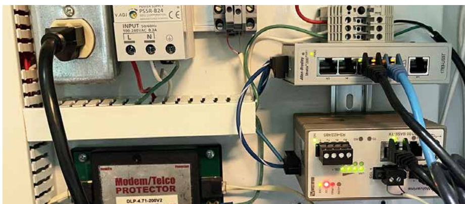
Wolverine line extenders (bottom right) remove the need to install new fiber optic cabling.
