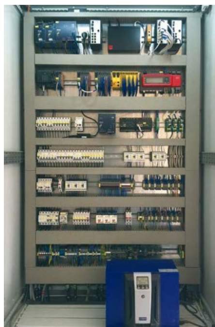
Control cabinet for energy management and battery control system – featuring a controller, safety components and SiteManager.
