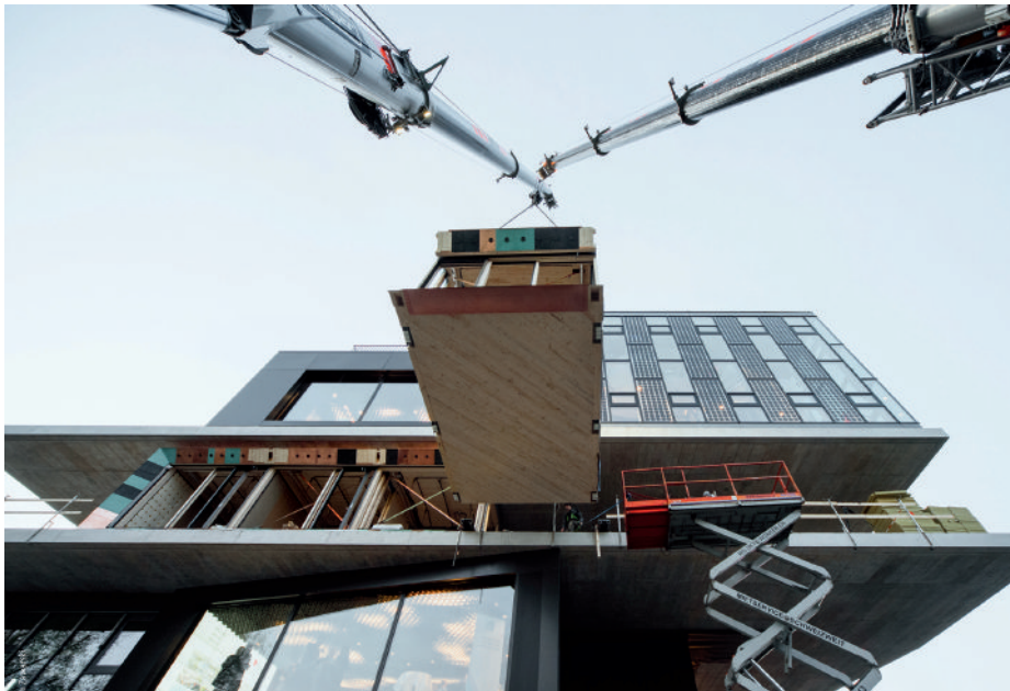
Research units can be added to NEST easily using a large-scale plug-and-play principle.
